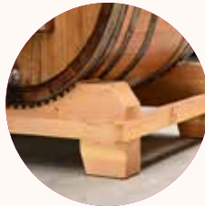
Replacement of barrel racks
