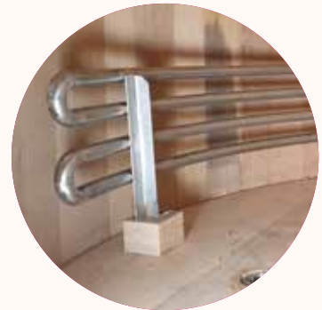
Cooling plates and cooling coil
